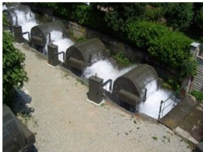
Fig. 2- activated water wheels
