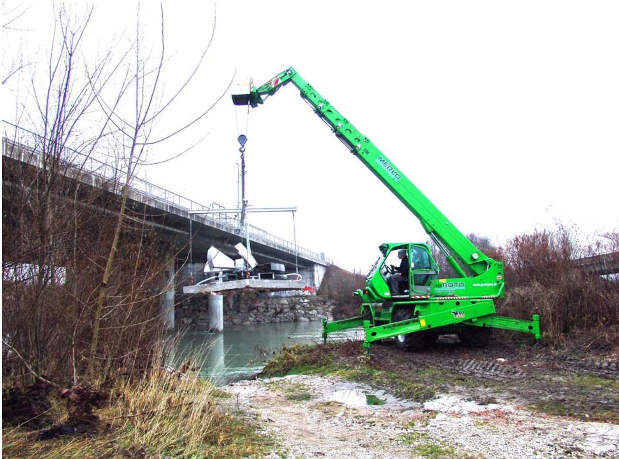
Picture from October 2009<sup>th</sup> year: Smaller unit SP 1 on a concrete basement plate, during assembly on the bottom of a slow river stream near Ljubljana.
