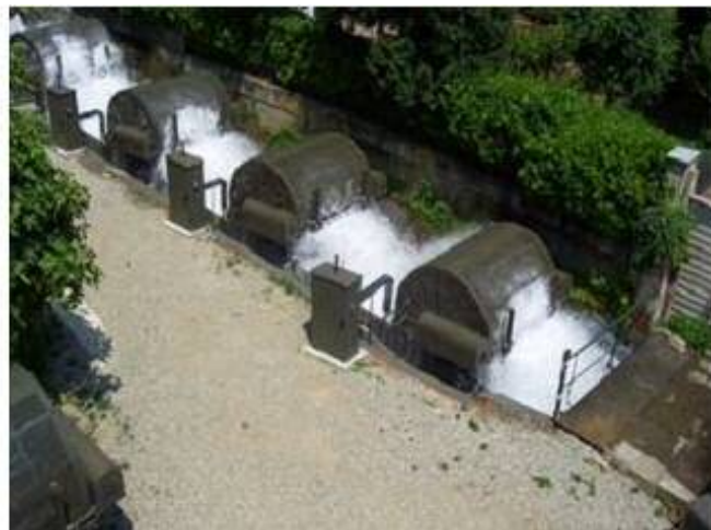
Fig. 2- activated water wheels
