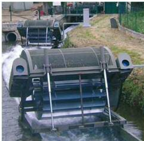
Fig.1-water wheels during maintenance
