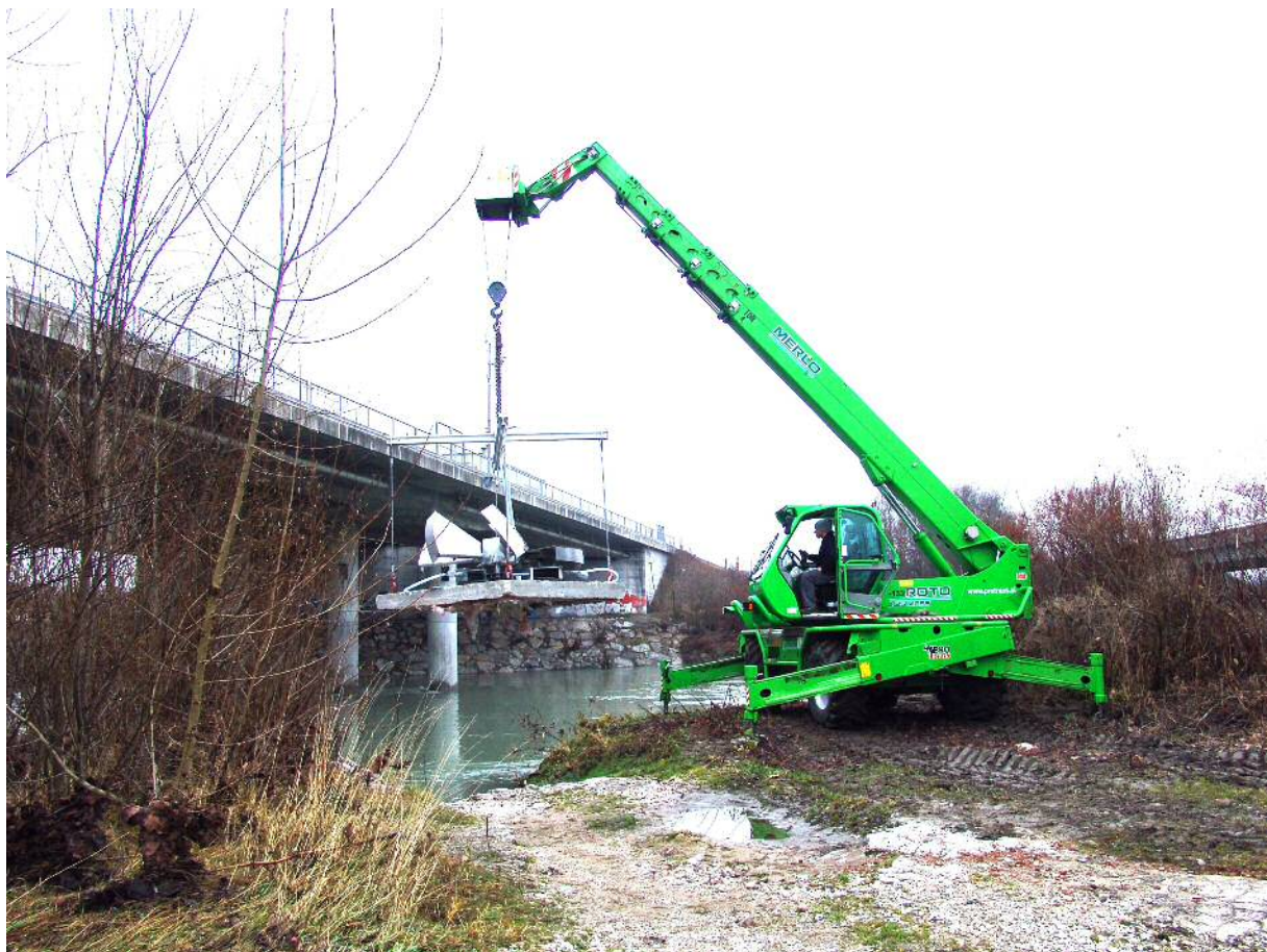
Picture from October 2009 th year: Smaller unit SP 1 on a concrete basement plate, during assembly on the bottom of a slow river stream near Ljubljana.
